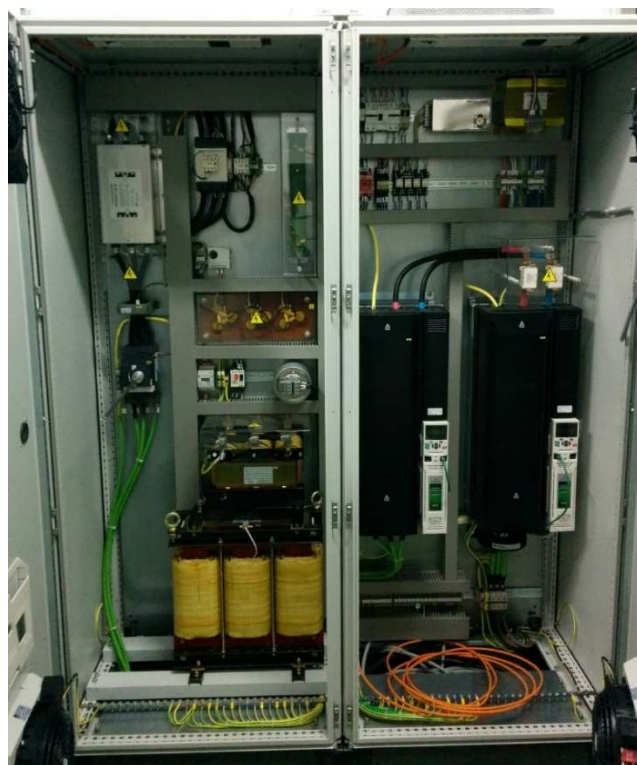
FIGURE 5. INTERIOR VIEW OF POWER ELECTRONICS CABINET
