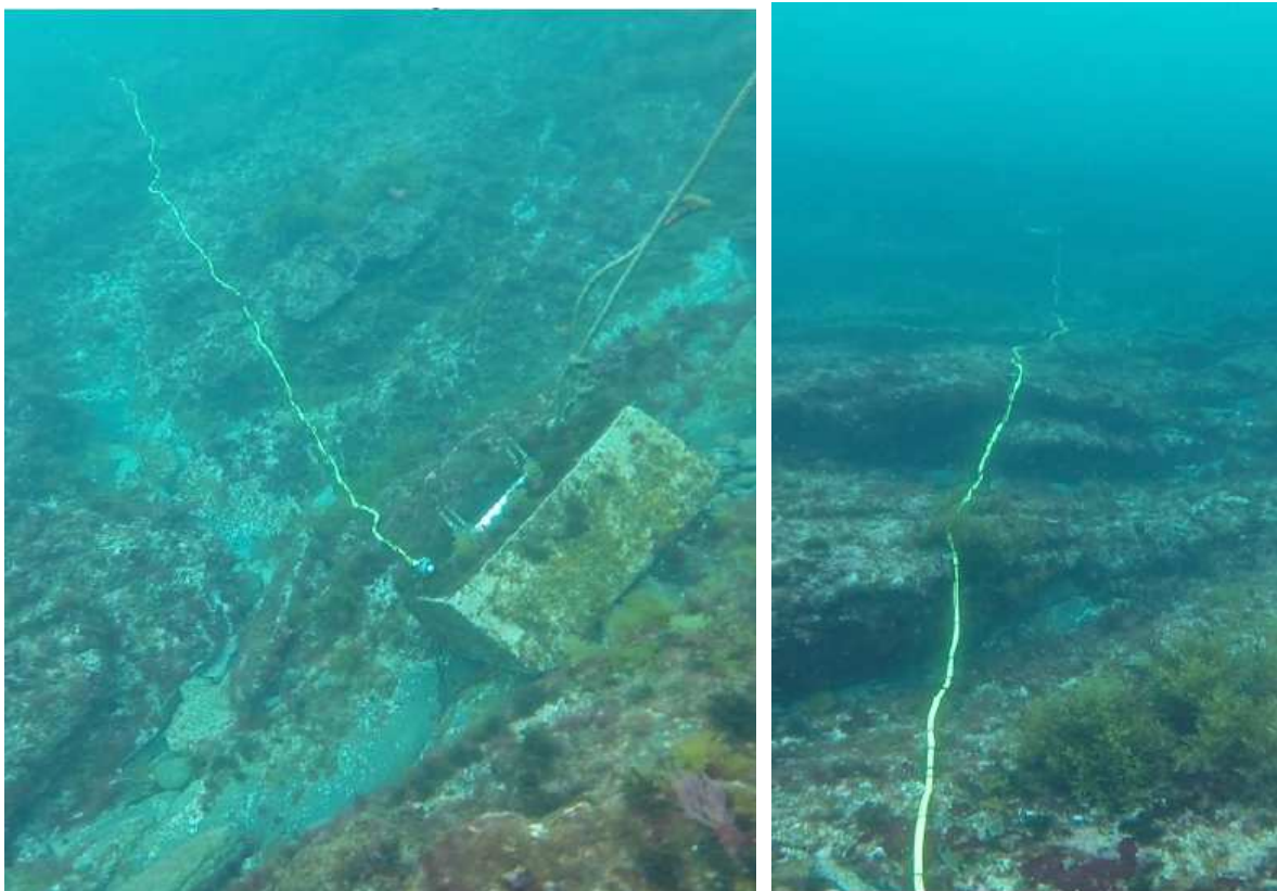
FIGURE 2. CNC4200 AND COMMUNICATION CABLE INSTALLED AT SUBSEA
