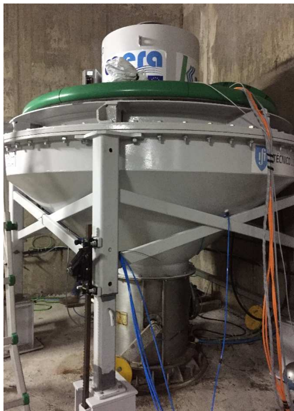
FIGURE 3. TURBINE INSTALLED IN MUTRIKU WAVE POWER PLANT
